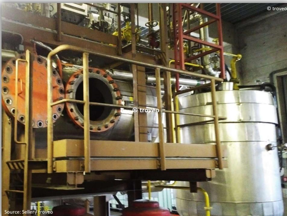
flue gas cleaning system - ammoniac evaporator station for the DeNO<sub>x</sub> filter
