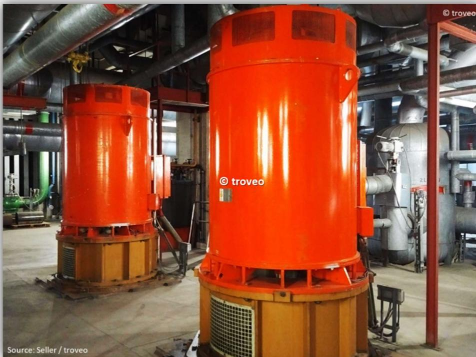
water/steam cycle – main high-pressure condensate pumps
