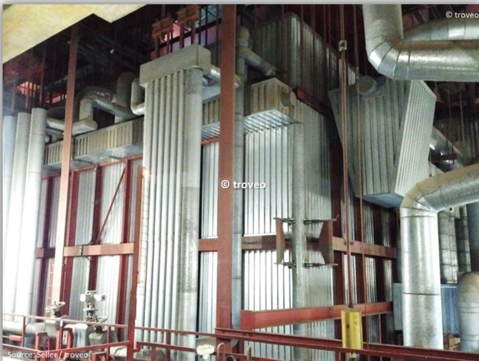
steam boiler – boiler top-side suspension
