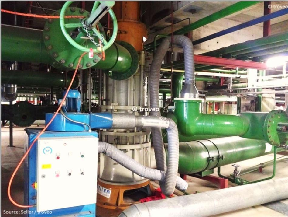
water/steam cycle – one of more than 40 fan air heaters/dryers,
