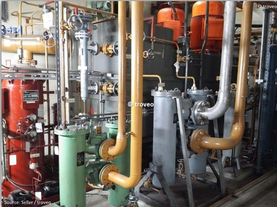
steam turbine – bearing oil lubrication system
