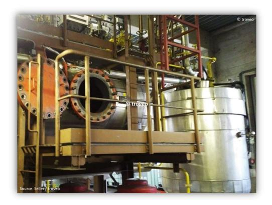
flue gas cleaning system - ammoniac evaporator station for the DeNOx filter
