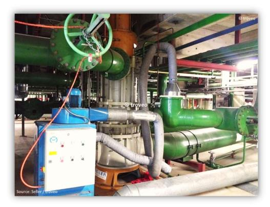
water/steam cycle – one of more than 40 fan air heaters/dryers, temporarily installed for plant preservation
